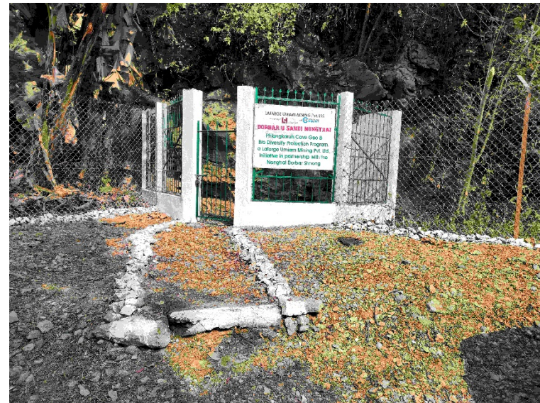
Fencing around Cave Area for its Protection.
