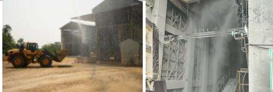
Water Sprinklers in Dump Hopper and Rain water Gun for water sprinkling in the surrounding area
