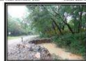
Check dam to South of the Mine
