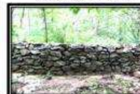
Check dam to Southeast below PWD Road
