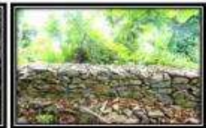
Check dam to Southeast of the mine
