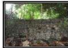
Check Dam near Transit House
