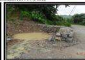
Check dam to Southwest of the Mine
