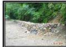
Check dam near Mine Entrance Gate
