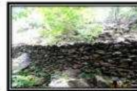
Check dam to West of the Mine
